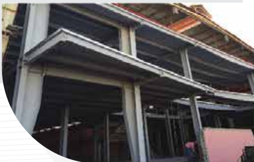
AL WATANIYA STEEL LABOUR CAMP
