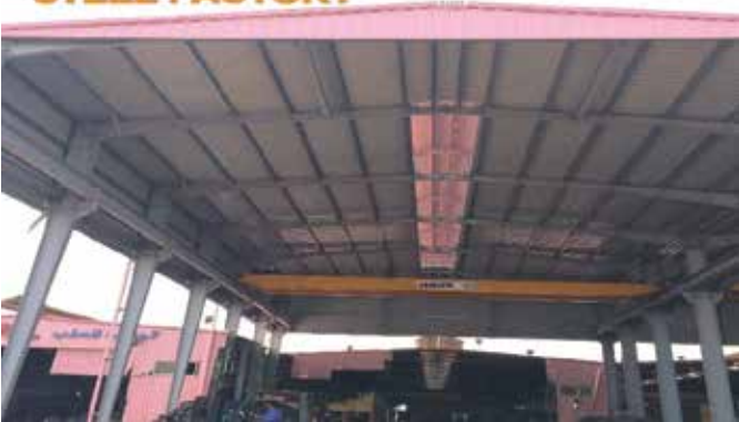
AL-WATANIA STEEL FACTORY
