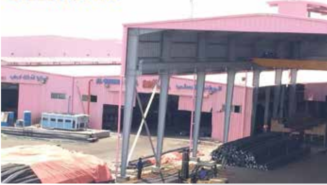
AL-WATANIA STEEL FACTORY
